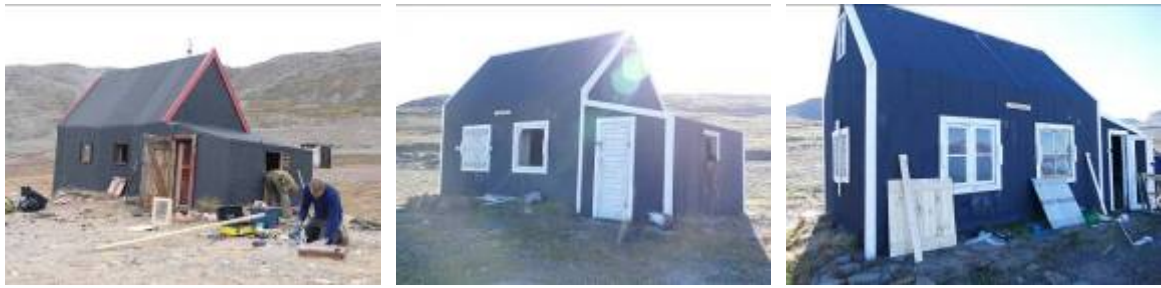
Left: Repairing Kap Humboldt [308]. Middle and right: Laplace [301] before and after.
