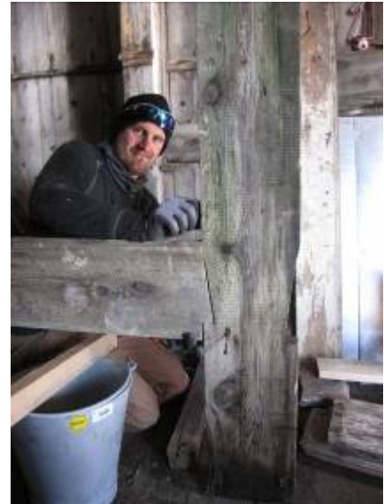
On the east wall, the freestanding pillar by the bunks' bearers was a mystery. The two east-facing bunks' bearers were attached in some characteristically recessed fenders. On the other side of the pillar there were identical fenders.
