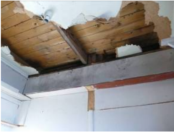
Left: In several of the rooms in Ørnereden the bear had destroyed the ceiling plates in 2013.
