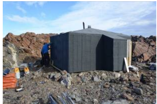
Walls and roof were covered with inner roofing felt, which was nailed on with 25 mm roofing nails. 18,000 roofing nails in total with 5 cm in between.
