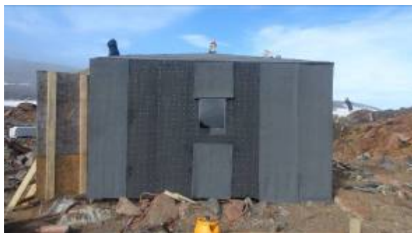
The outer roofing felt was melted on with overlaps considering water from above and the predominant wind directions (NE and SW).
