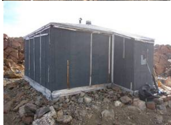
On the roofing felt of the walls the original fillets etc. were attached precisely where they had been installed previously.
