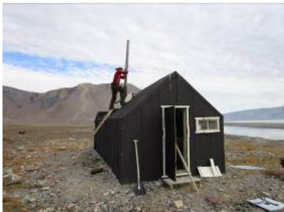
Left: New stovepipe on Strindberghuset [358-3]. Right: Emergency repair of stovepipe on Nordfjordhuset [358-2].
