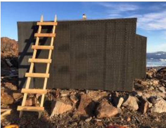
Walls and roof were covered with inner roofing felt, which was nailed on with 25 mm roofing nails. 18,000 roofing nails in total with 5 cm in between.
