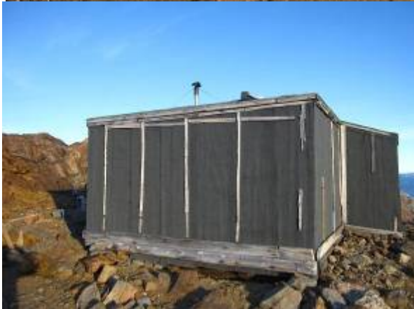
On the roofing felt of the walls the original fillets etc. were attached precisely where they had been installed previously.
