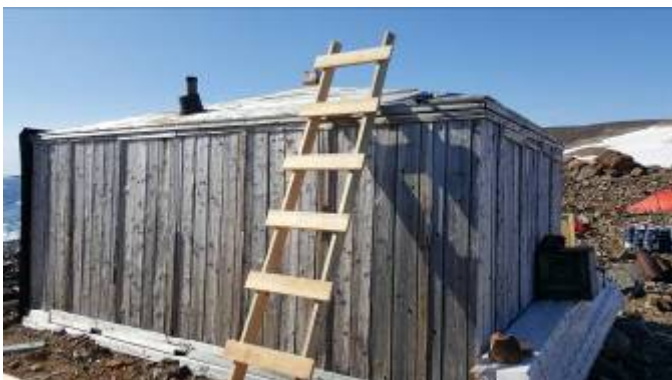
All of the roof boards were re-nailed so the roofing felt was not put on an unstable base.
