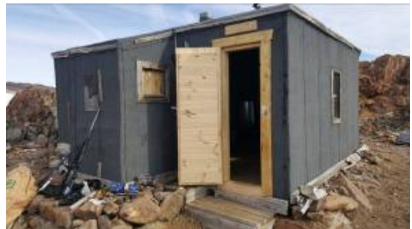
The outer roofing felt was melted on with overlaps considering water from above and the predominant wind directions (NE and SW).
