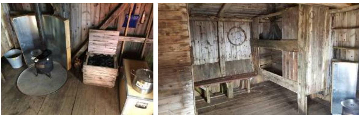
The round shape of the cover plate called for a similar round reflecting screen which was produced from the materials in which the Nanok stove had been packed.
