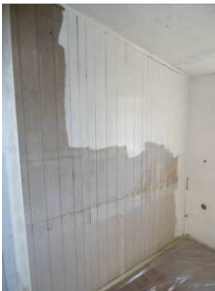
Tolvmandsbarakken was painted inside from floor to ceiling. It takes time, but it is worth the while. In the middle the central coal stove of the barracks can be seen.
