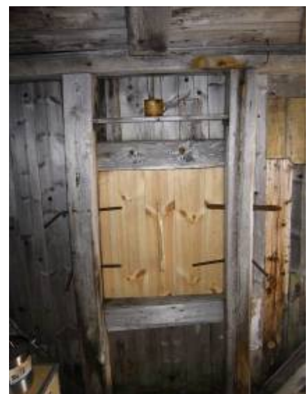
Because of the visits from the bears, we decided to produce shutters for the windows to improve the bearproofing of the hut. We installed the shutters on the inside to keep the original appearance outside.
